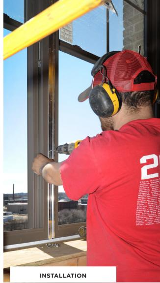
Receptor systems have long been used on job sites with aluminum windows, but now there is a customized solution for vinyl window projects. Harvey's aluminum receptor system **simplifies and accelerates installation** in projects with challenging existing conditions. This thermally broken product is used in place of interior/exterior stops, resulting in a cleaner look than traditional installations.
